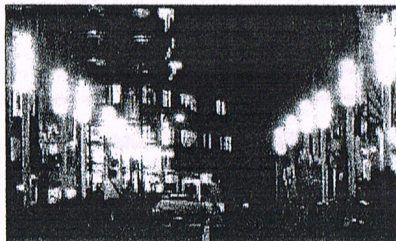
Installation of street lights
